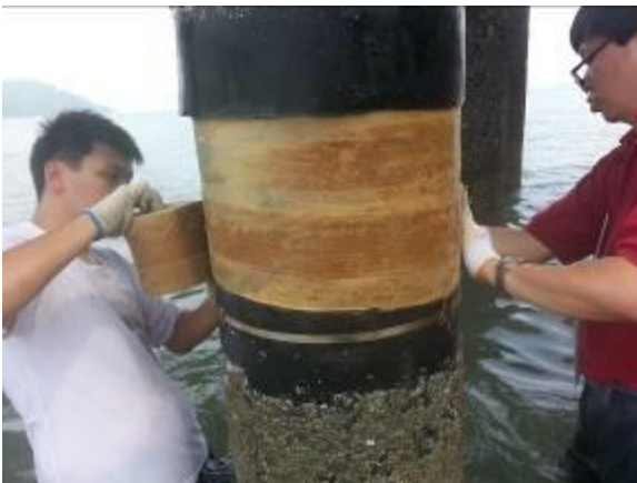
Photo 36: Apply 2 layer STACwrap
