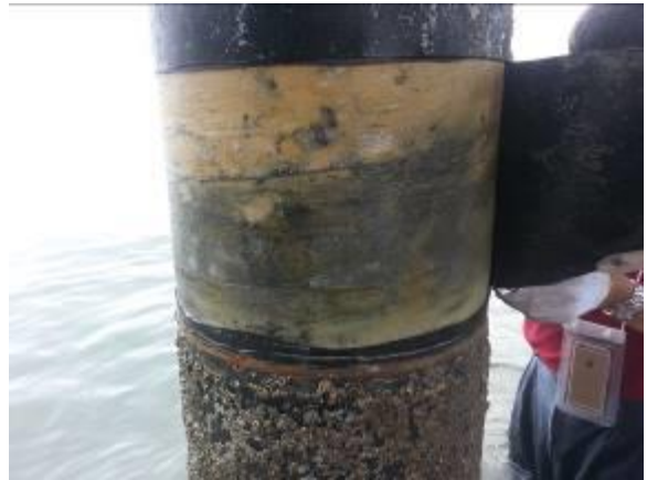
Photo 28: Condition of STACwrap
