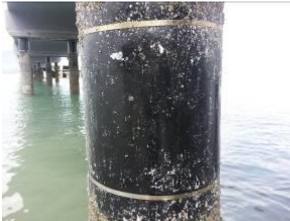
Photo 21: SS317L Strap Removed
