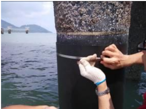
Photo 42: Install Top SS317L band
