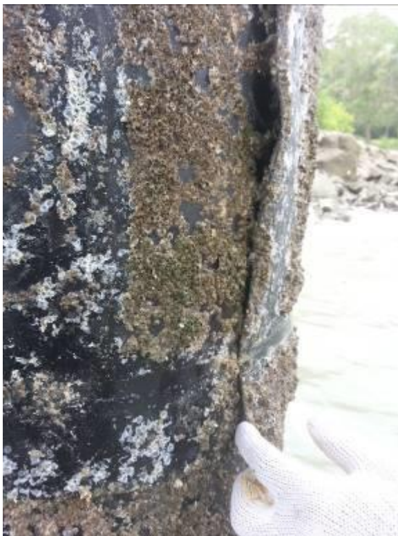
Photo 21: SS317L Strap Removed
