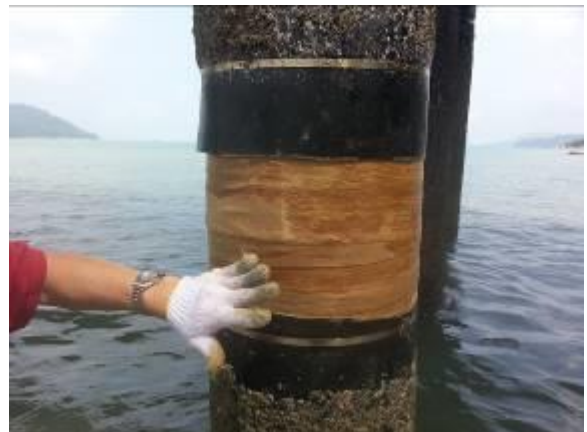
Photo 39: Complete 2 layer STACwrap
