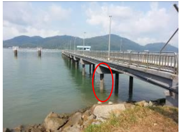
Photo 16: View of Selected Pile
