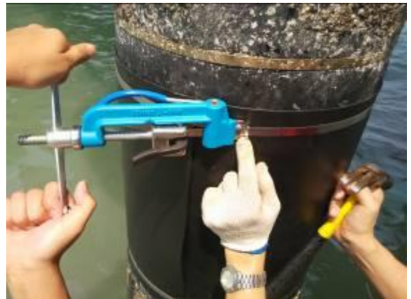
Photo 43: Install Top SS317L band
