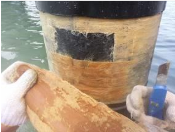
Photo 34: Patch with STACwrap
