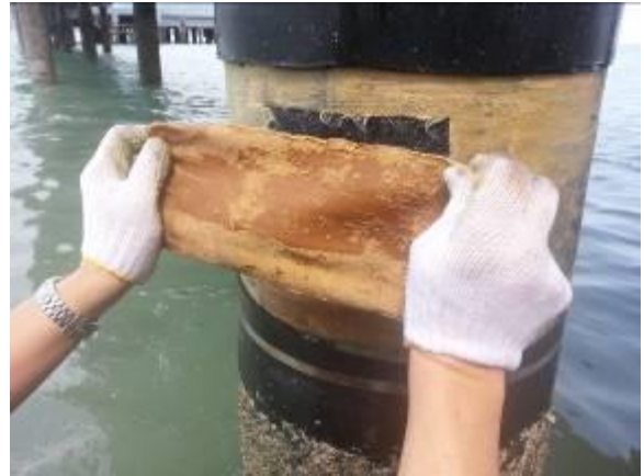
Photo 35: Patch with STACwrap
