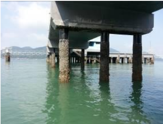
Photo 5: View of Trestle
