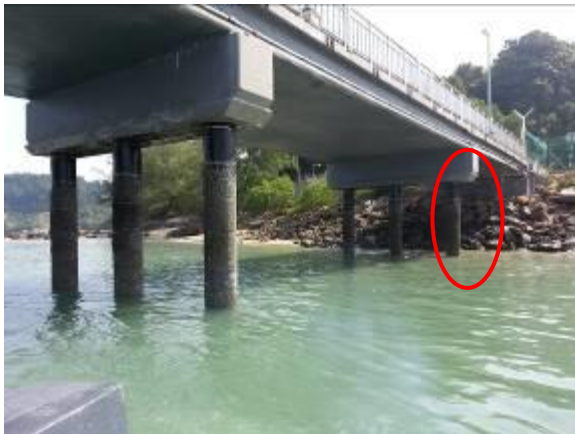
Photo 15: View of Selected Pile
