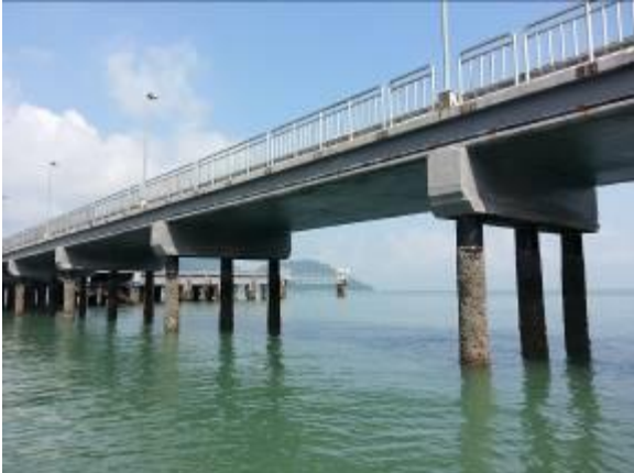
Photo 7: View of Jetty
