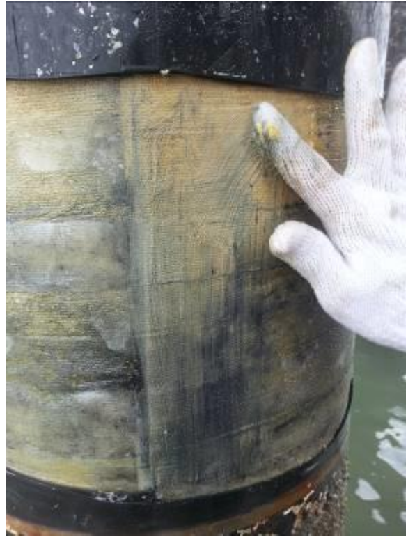
Photo 26: Condition of STACwrap
