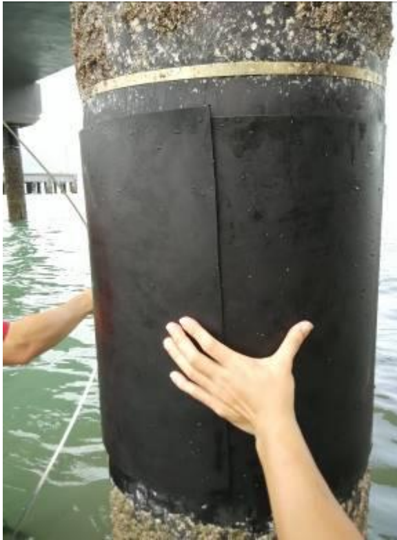
Photo 40: New Section of Jacket
