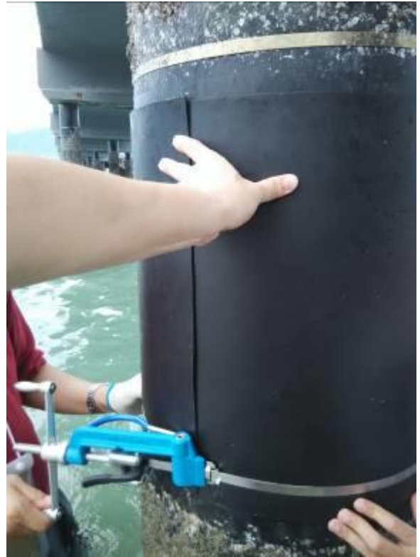
Photo 41: Install Bottom SS317L band
