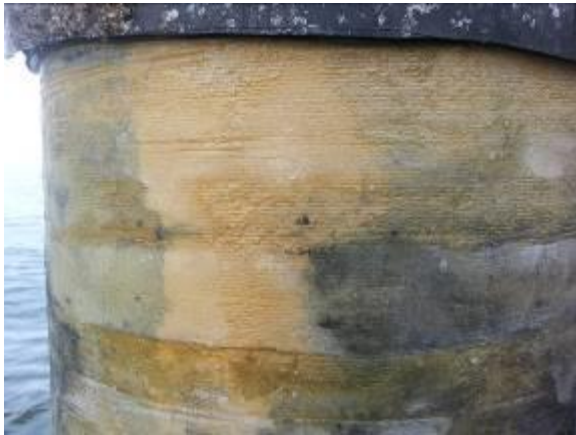
Photo 27: Condition of STACwrap
