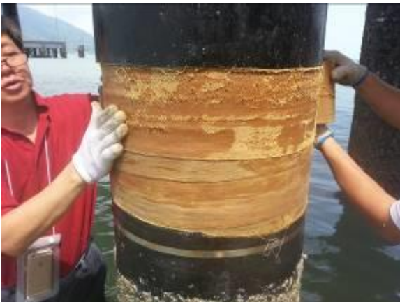
Photo 38: Apply 2 layer STACwrap
