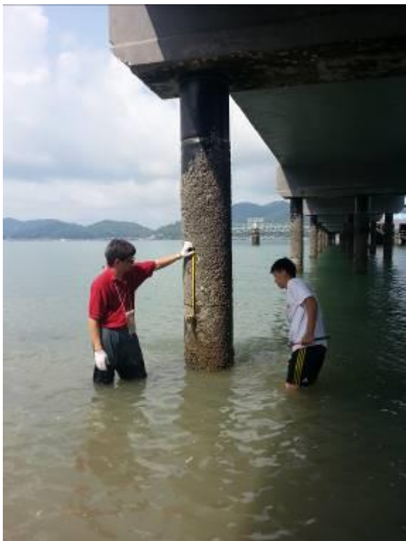
Photo 17: Inspection of Pile
