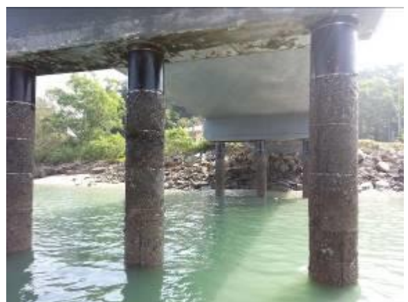
Photo 6: View of Trestle
