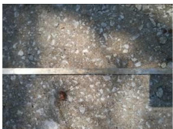
Photo 50: The removed SS317L bands
