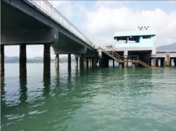
Photo 8: View of Jetty
