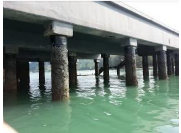
Photo 4: View of Trestle
