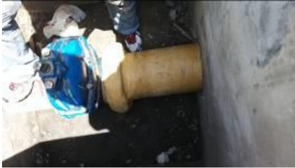
Photo 13 : View after apply STACwrap
