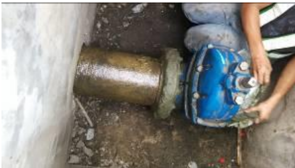
Photo 09 : View after apply STACfill
