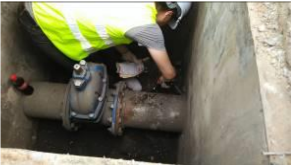
Photo 04 : Cleaning with hand tools
