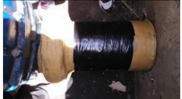
Photo 14 : View after apply STACguard
