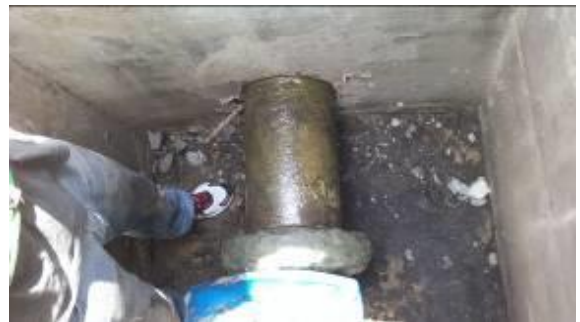
Photo 10 : View after apply STACfill
