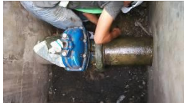
Photo 08 : Apply STACfill on flange area
